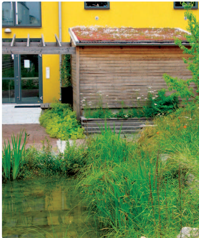
Fig. 2 A storm water pond in a courtyard at Bo01, Western Harbour, Malmö - the pond is built as a semi-natural biotope with regional wetland plants; in the background is a green roof, with edge of a woodland on the right
