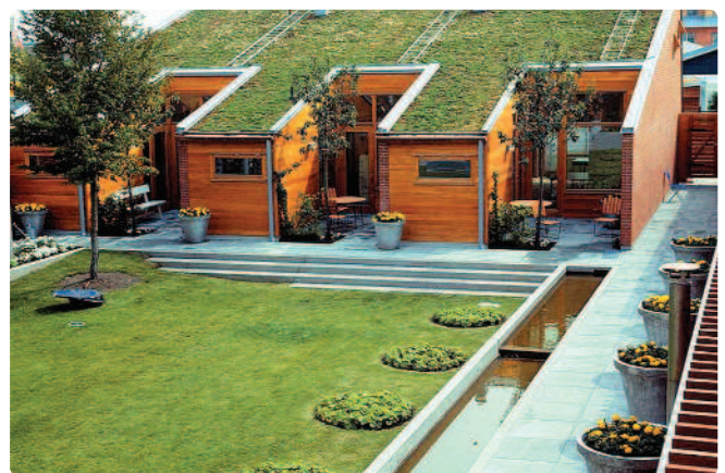
Fig. 4 The courtyard with the highest Green Space Factor (a score 0.84) at Bo01, Western Harbour, Malmö achieved its rating mainly with mown lawns and sedum roofs
