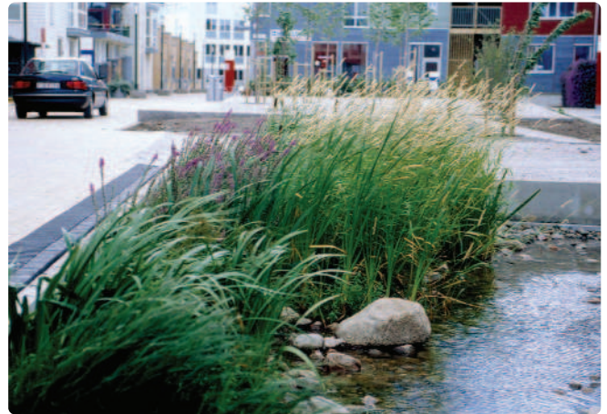
Fig. 1 Vegetated ponds form an important part of the stormwater system at Bo01, Western Harbour, Malmö
