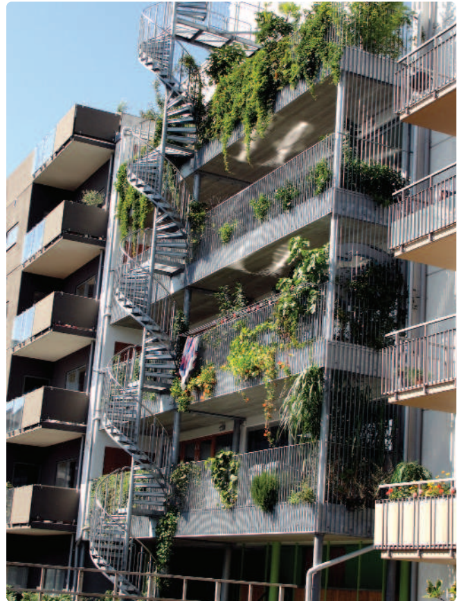
Fig. 7 In the 'Urbana Villor' project the large balconies have 300 millimetre substrate covering the whole balcony area. A system of tiles makes it possible to use as little or as much as one wishes for vegetation, but the roots have large volumes of substrate. The balconies are not attached to the wall, but to a free-standing structure to avoid humidity problems
