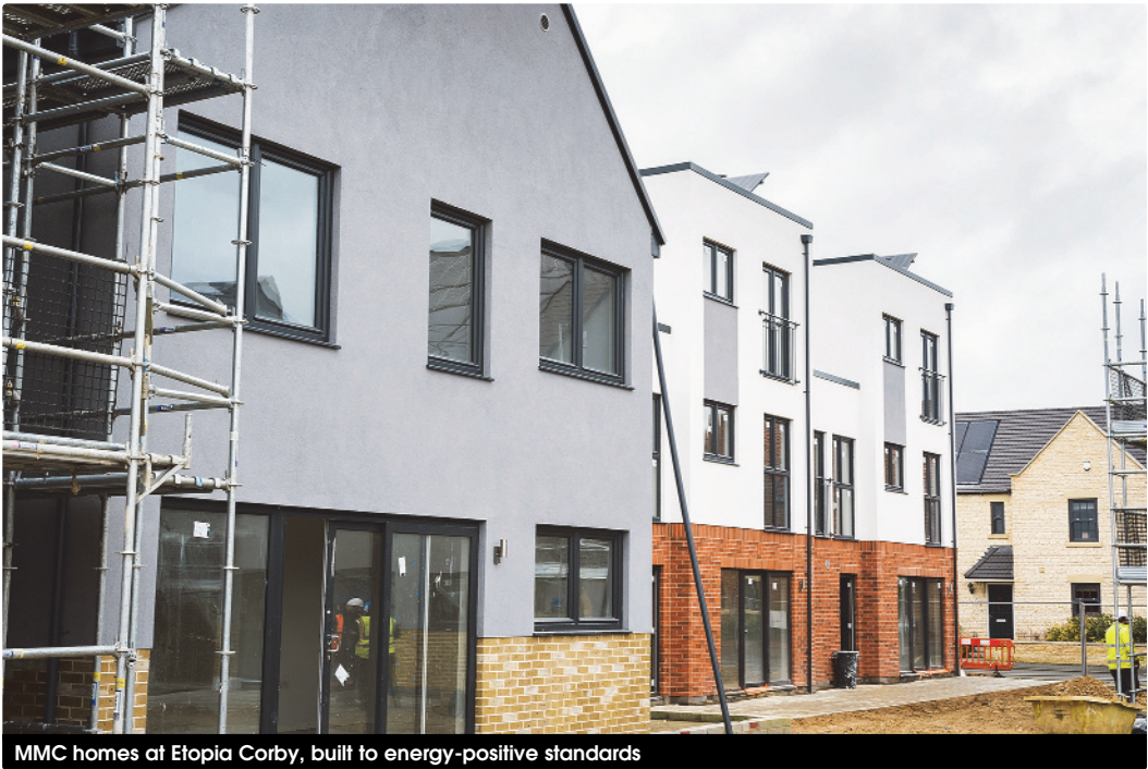
MMC homes at Etopia Corby, built to energy-positive standards
