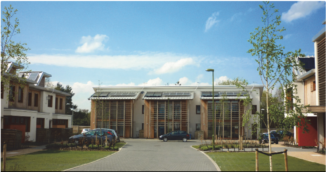
Integrating solar photovoltaic installations with the building fabric in Letchworth Garden City
