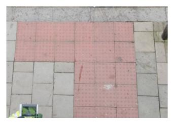
Tactile paving should be provided at all designated crossing points (using blister paving), to allow for the crossing to cover two strides and be physically detectable (note that the image illustrates national best practice and is aligned with DfT's Guidance on the use of tactile surfaces).
