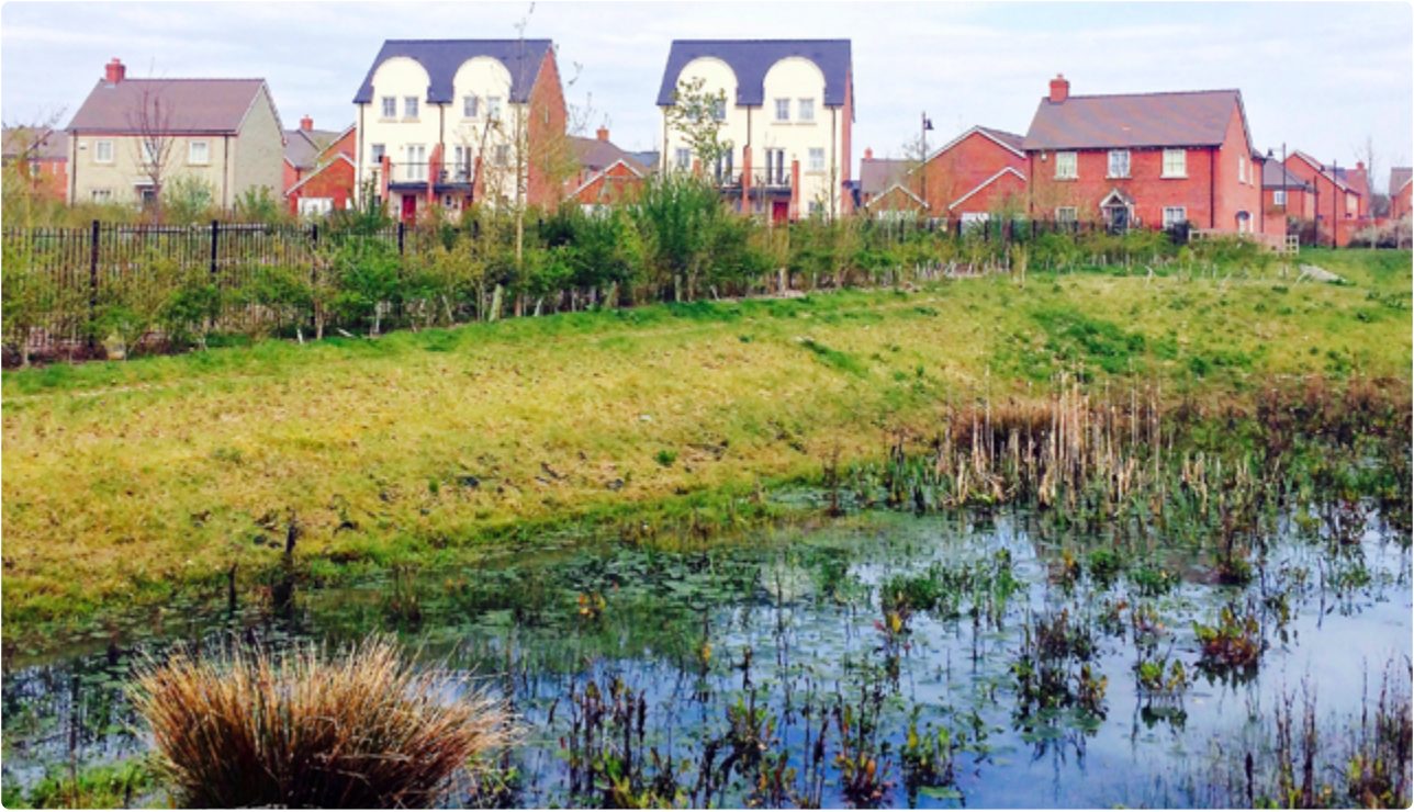
Sustainable urban drainage system associated with a new housing development
