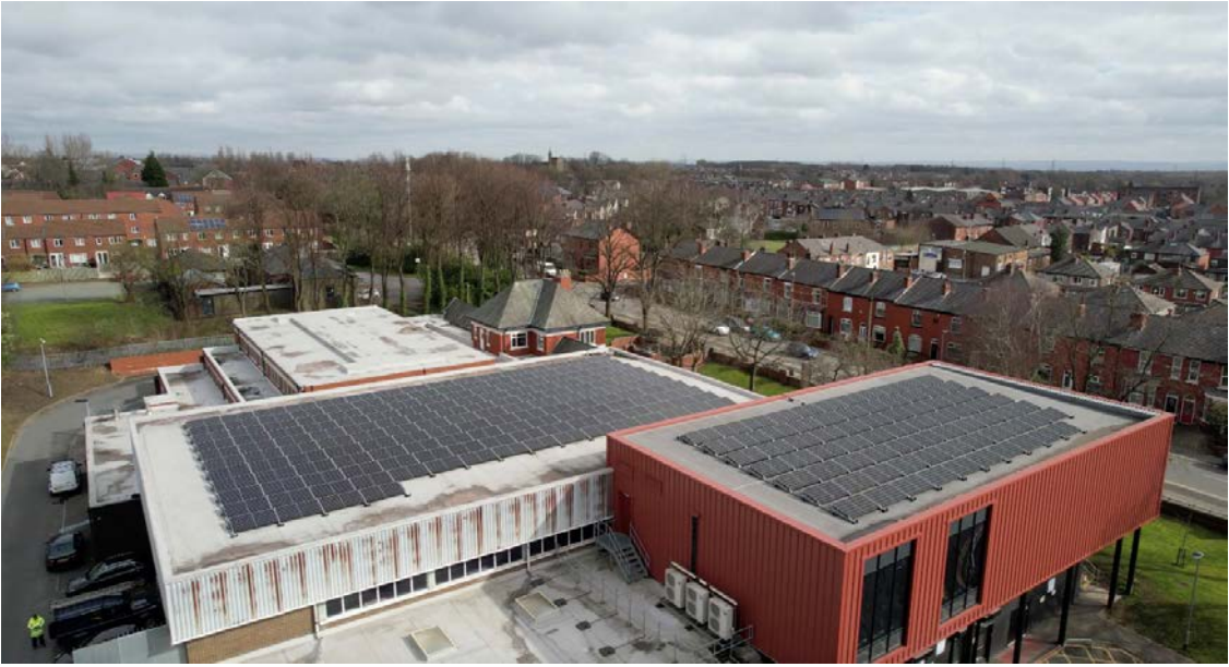
Figure 16: Solar panels installed on Worsley Leisure Centre, Salford. Source: Ben Nuttall, NPS Energy.
