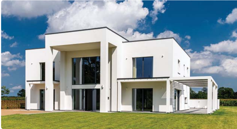
One of the grand Passivhaus Plus homes in Norfolk
