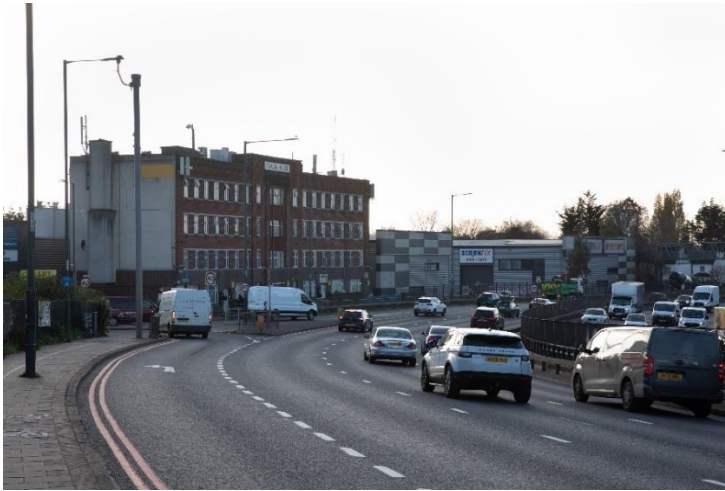
Figure 2. Beacon House, Neasden, London – PD converted flats facing the North Circular Road
