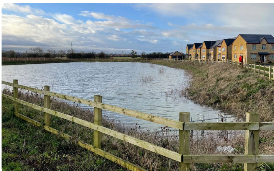
Image 2: SuDS attenuation pond holding water following heavy rainfall in January 2024. Source: JW Redfern, Twigworth Parish Council.
