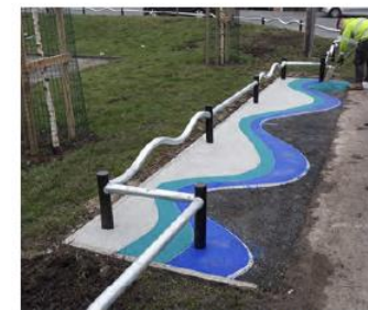
A colourful surface treatment being installed alongside wavy railings provides a 'playlet' for doorstep play along the Canterbury Estate school route. (Photo © Better Start Better Place)
